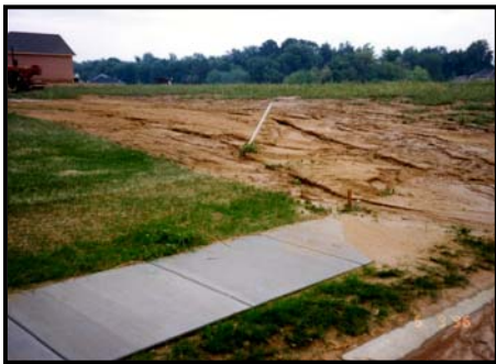
No erosion control
