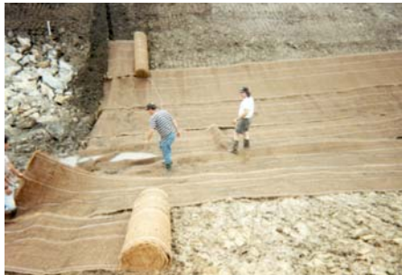
Figure 10. TRMs are easily installed without the need for heavy equipment (Images in order from left to right. A TRM being installed in a channel. The same channel after vegetation establishment).
